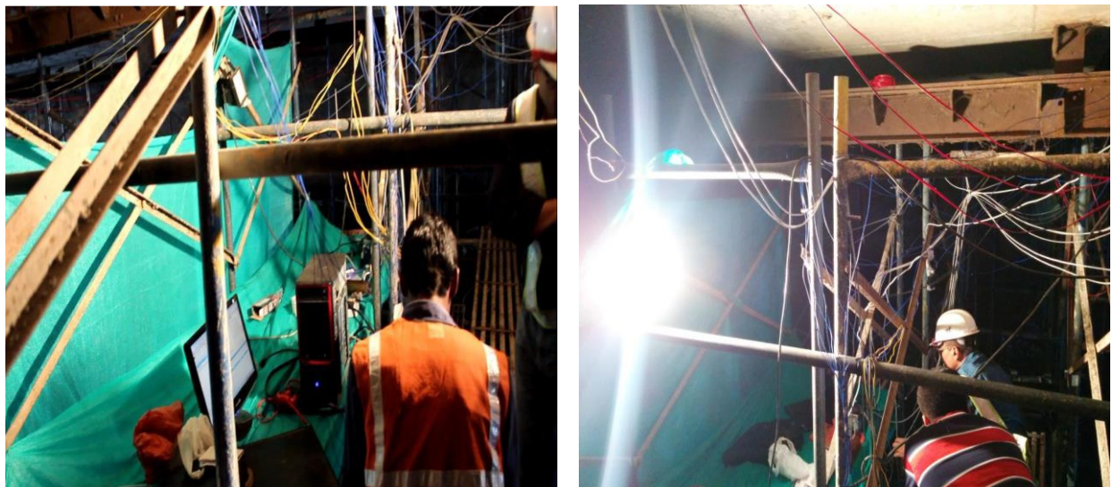
Figure 5. Wiring of Sensors near Data Acquiring Arrangement in Congested Site Area
