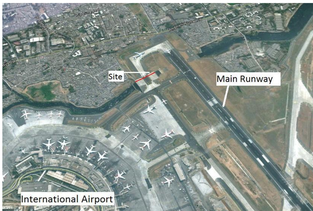
Figure 2. Position of Mithi River Bridge below the Runway
